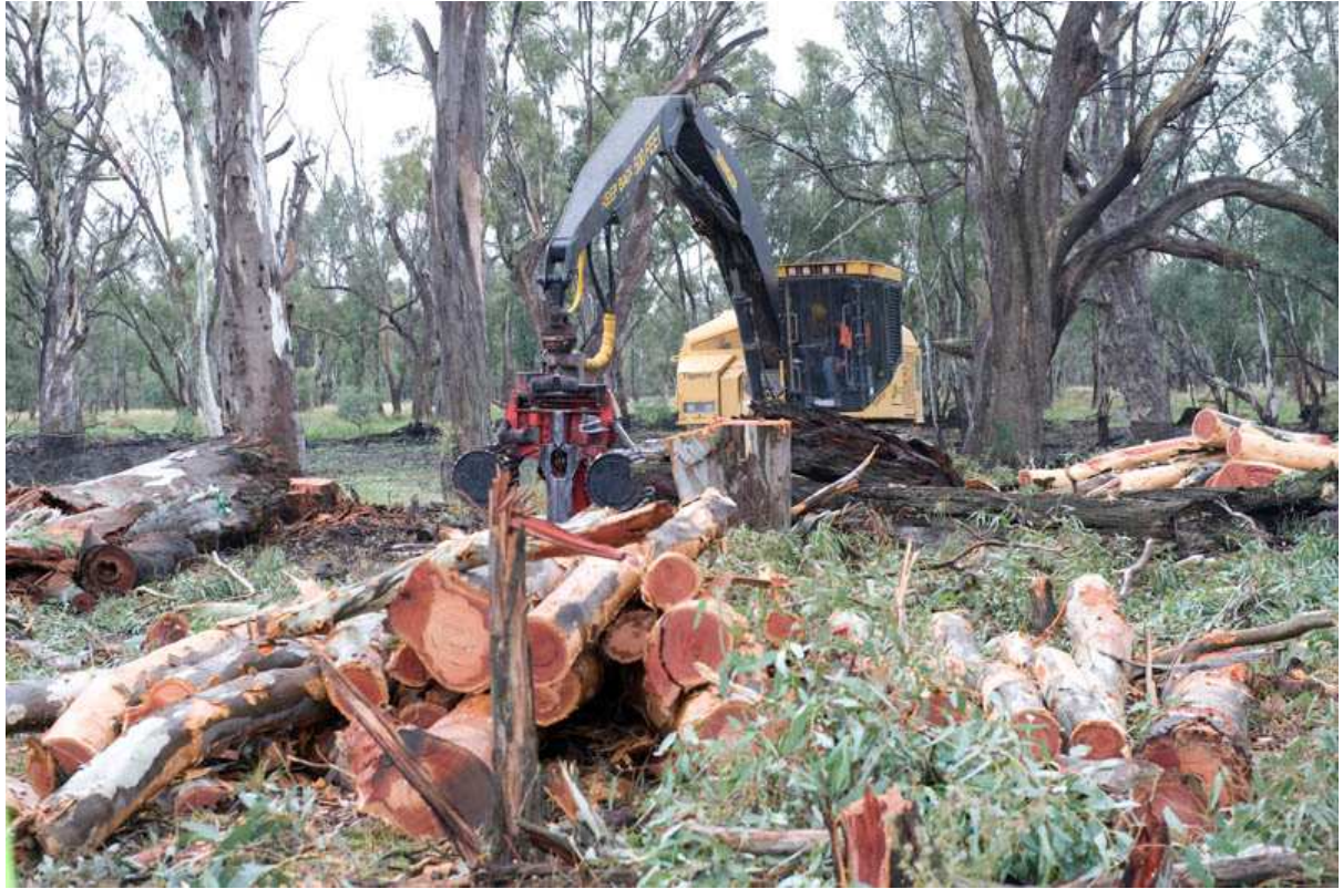
Harvesting in the levee footprint near Barham
