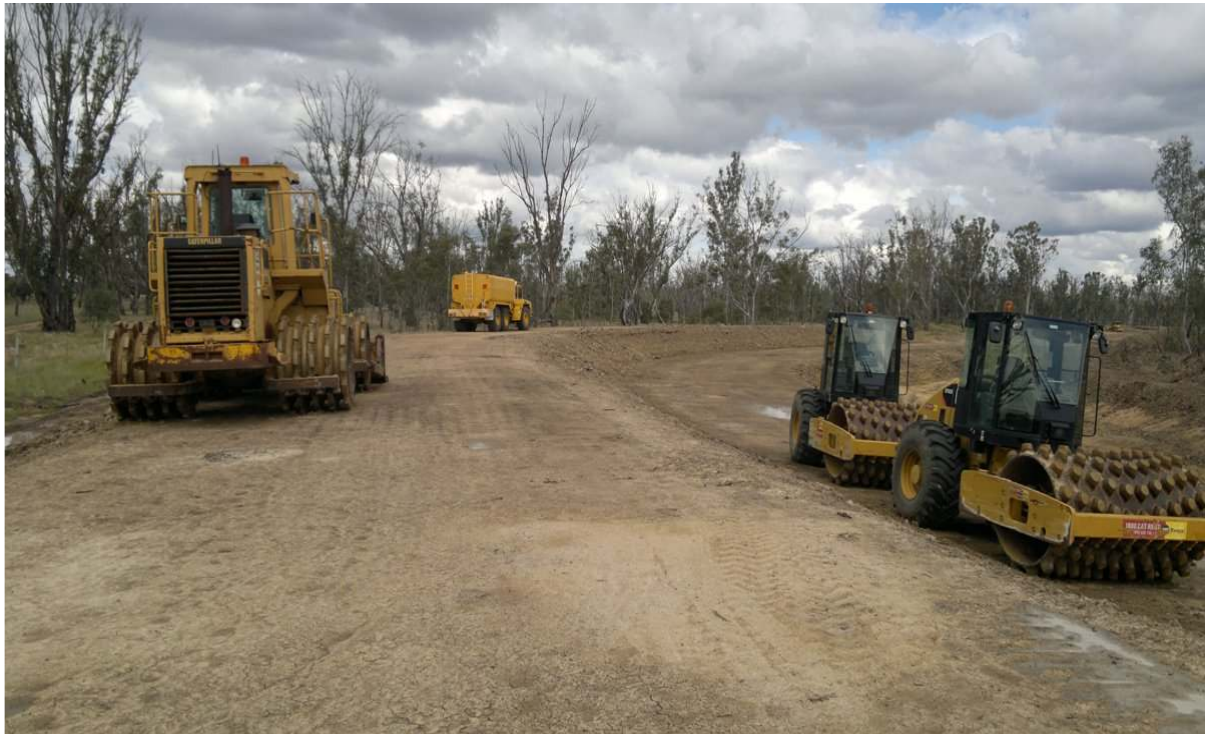
Levee construction works. Photo courtesy of Professional Engineering Services.
